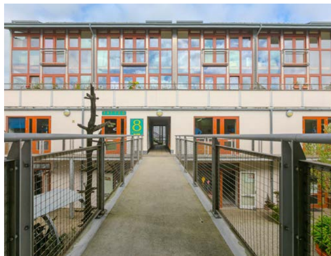
Link Bridge with residential apartments above workshops
